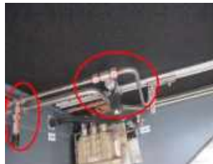
Sealing of air compressor tubings
